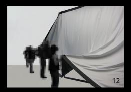
**10-12** Unroll the projection surface with, according to the screen size appropriate number of people and hook it onto the rail of the upper horizontal frame section and slide it with several people gently till the opposite corner.
